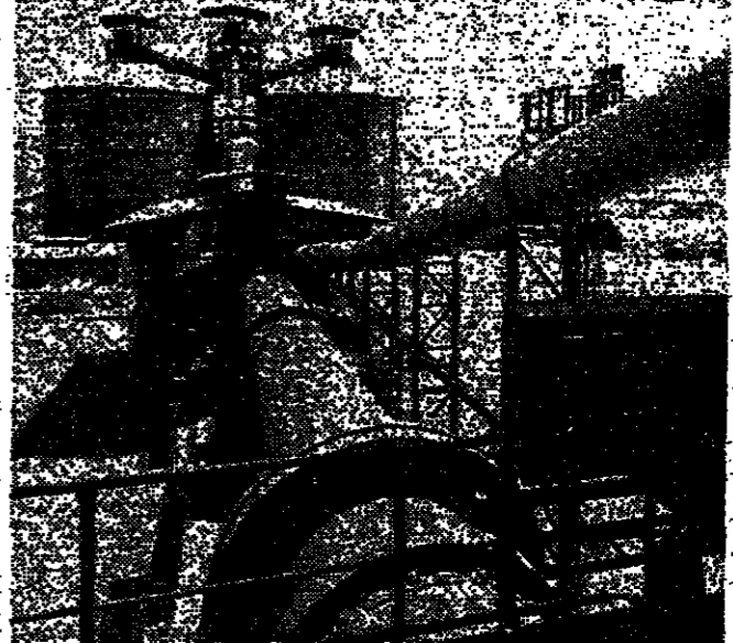
The new dry-process cement plant built by Costain International at Rusail industrial estate in the north. It and the new Mina Raysut factory will produce 60 per cent of Oman's yearly cement requirements.
